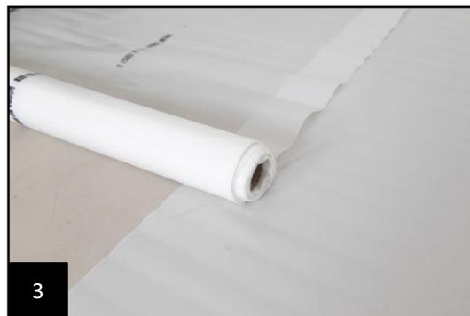
Then use the footfall and walking sound reducing insulation underlays recommended by Windmüller. For floor coverings with a laminated insulating carpet pad, also proceed as described above. Insulation underlays reduce sound transmission to other rooms, reduce footfall noise and thus significantly improve living comfort. The CS value (compressive strength) of insulation underlays should be at least  $\geq 90\text{ kPA}$ .
