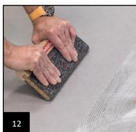
In order to achieve an optimum installation result, the covering must be carefully rubbed from the centre to the sides immediately after it has been placed (11) in
