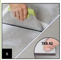
Now apply the adhesive approved by Windmöller GmbH evenly and lane by lane according to the adhesive manufacturer's instructions using the TKB toothed strip (usually TKB A2 toothing) recommended for this purpose (8).
