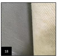
Afterwards, but not later than 30 minutes after manual rubbing, the covering is evenly and slowly rolled (17) using an articulated roller (weight min. 50 kg / 110lbs). Check that the covering is sufficiently wetted (18) with adhesive.
